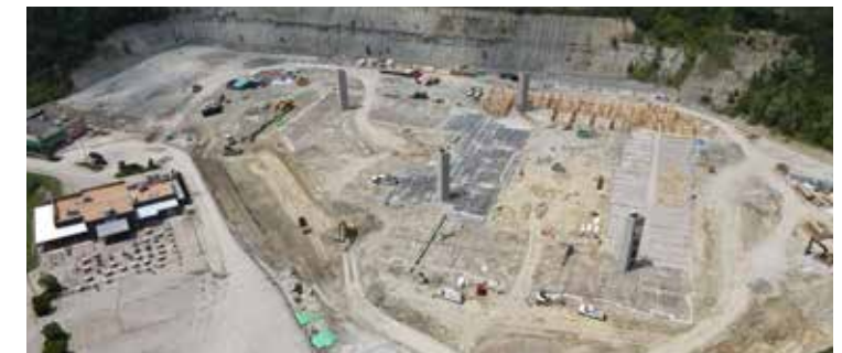
Future stairwells under construction at Skytop, a new apartment community.
