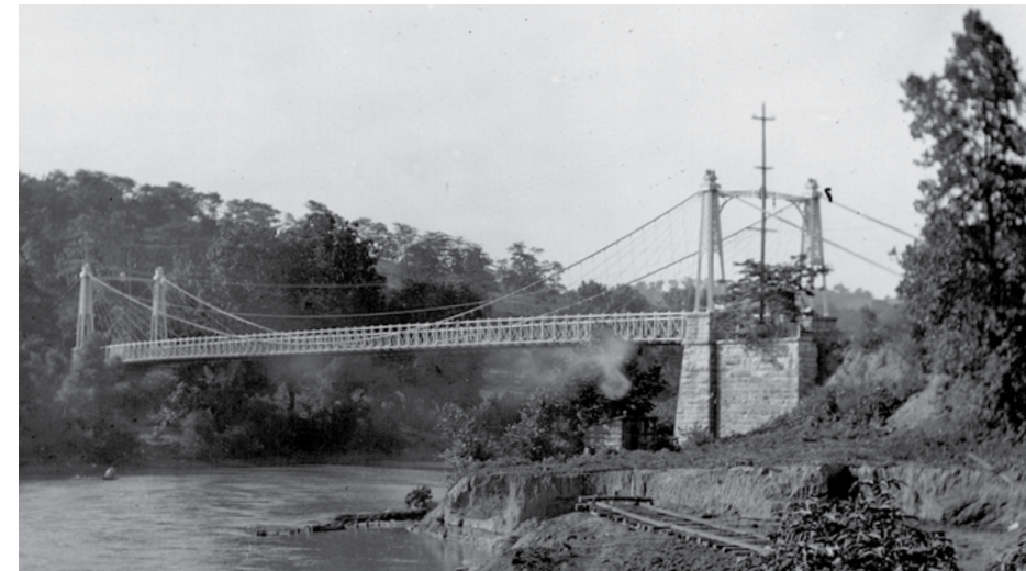
The suspension bridge over the Little Miami River at Beechmont Avenue, under construction about 1874.
