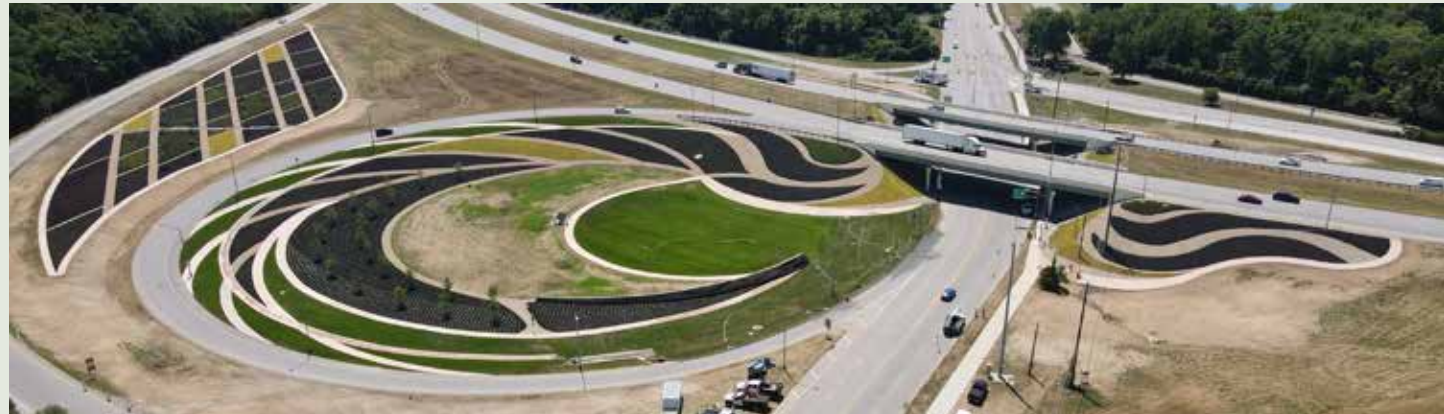
Aerial view of I-275 Exit 72 interchange project
