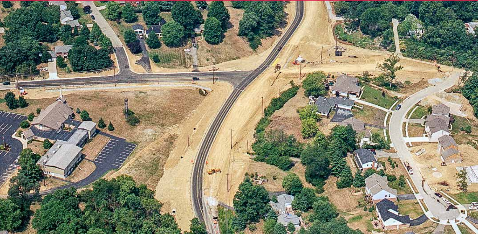
Previously, the Wolfangel intersection was offset which resulted in significant safety concerns. This project aligned the intersection with traffic signals, eliminating many safety issues. Photo courtesy of Henry Dolive.
