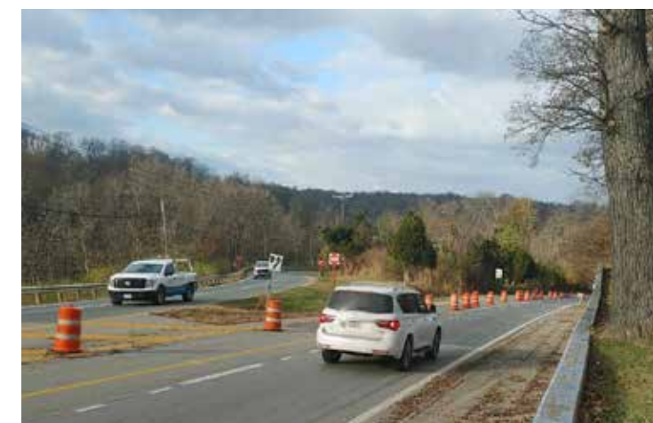
Construction started this fall on the S.R. 32 intersection upgrade.
