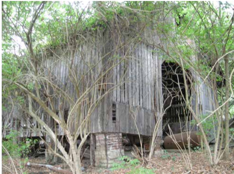
View of the corn crib in September 2007. When in use, it held about 7,000-9,000 bushels of ear corn. About 25 percent of the crib was salvaged for use in the History Room.
