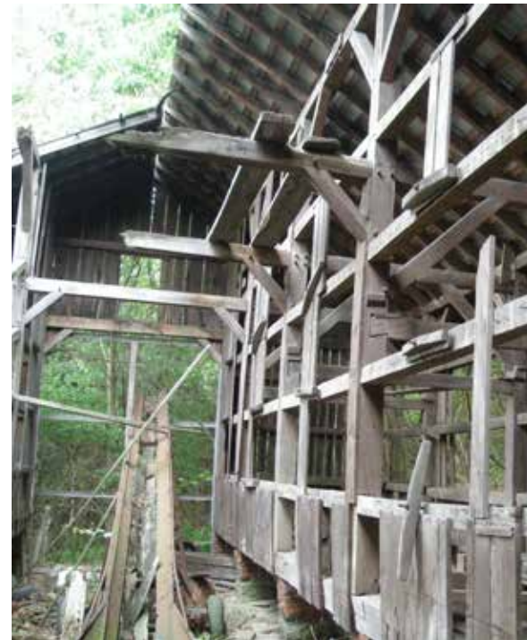
This interior photo from 2007 shows the post-and-beam structure of the crib, using one-inch in diameter hand-carved pegs.
