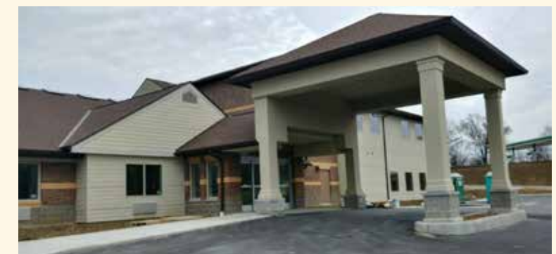
Forest Hills Care Center expansion
