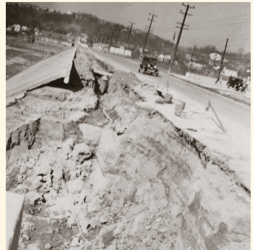
After the flood waters dropped, travel was restored across what is now called the Beechmont Levee along Lunken Airport. The image shows some of the flood damage. It is said that the 1937 flood gave rise to the airport's nickname “Sunken Lunken” and made clear the need for a new airport on higher ground.
