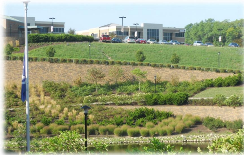
A stormwater management facility that is contoured to blend into the surrounding landscape.
